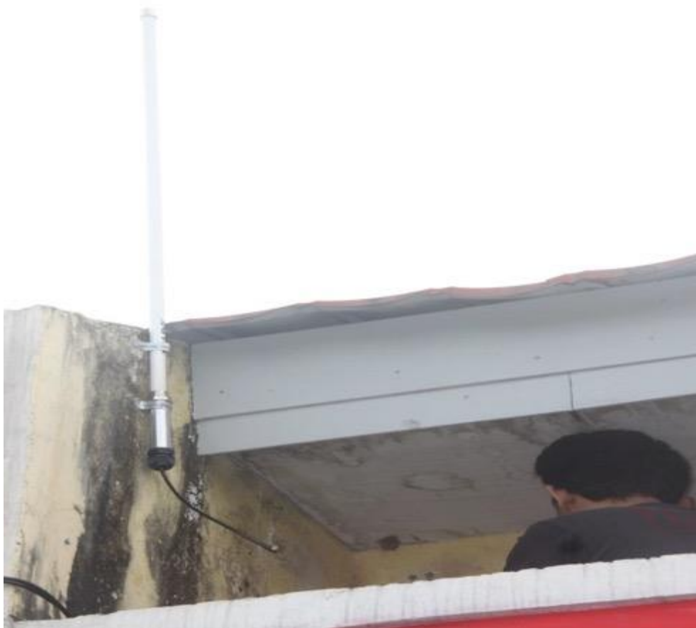
Gambar 4.36 Pemasangan Antena Omni (Wireless Outdoor)
