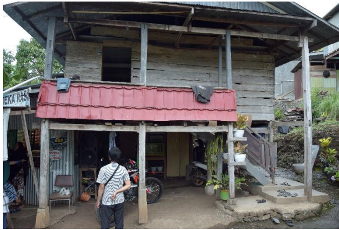
Figure 13: facade rumah L4
