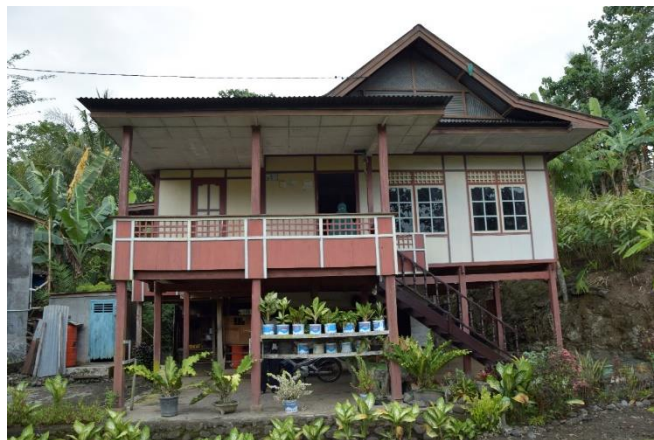
Figure 10: Facade rumah L3
