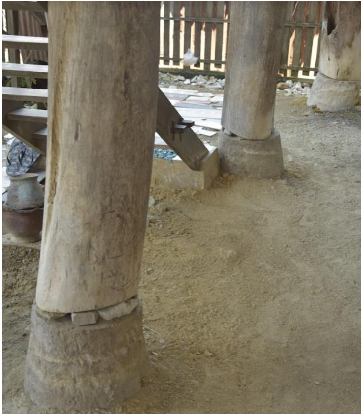
Figure 47 : T7 kolong, tiang berukuran Bundar, Sumber : Photographer Andi Abidah dan Taufiq Natsir
