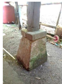
Figure 4 Pondasi Umpak
