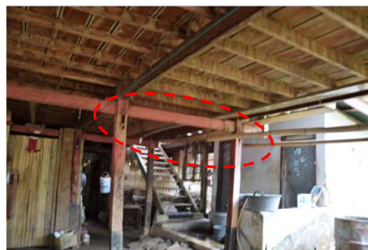
Figure 9 the hole as structure place old tamping model
