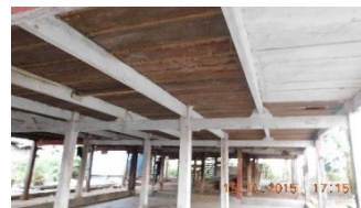
(b) the floor of the house with one big beam.
