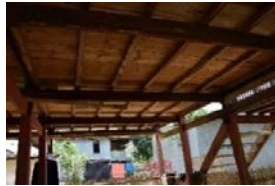
(b) floor of house. (the result of survey; 2015)
