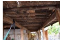
(b) the floor of the house. (the result of survey; 2015)
