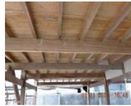
(b) the floor of the house, (the result of survey; 2015)
