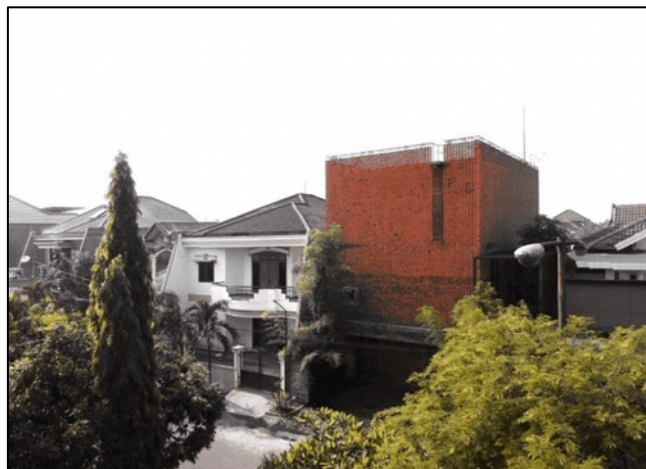
Fig. 1. Omah Boto Building Source: Wijaya et al. (2019)
