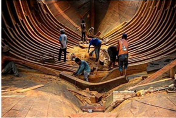
(a) Body Construction of Pinisi Vessel
