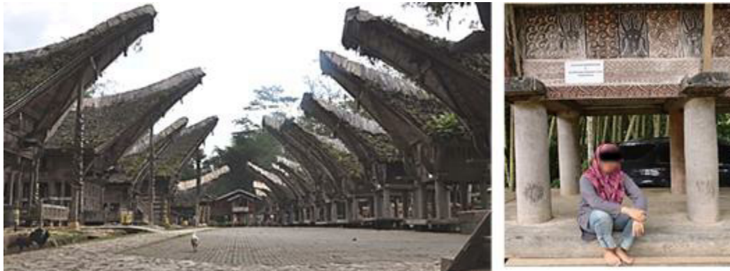
FIGURE 1. Traditional house (tongkonan) located at the opposite of the row of rice barn (alang sura) at Kete Kesu complex in North Toraja using wanga ( Pigafetta elata ) as building pole (Photo by Syamsiah)
