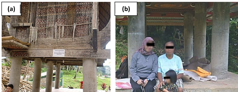
FIGURE 2. Model of rice granary (alang sura) using wanga ( Pigafetta elata ) in Tana Toraja Regency with different number of poles: (a) 8 poles and (b) 6 poles (Photo by Nani Kurnia and Eka Setiawan)
