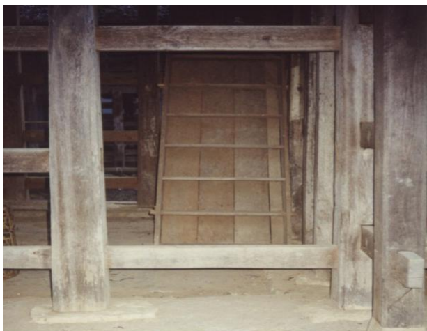
Figure 6. Photos showing the stairs below at Tongkonan Kesu '
