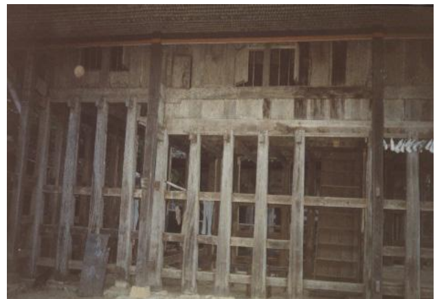
Figure 8. East side view of pole structure ( lentong garopang , lentong alla 'and roroan lambe ' ) at Tongkonan Kesu '
