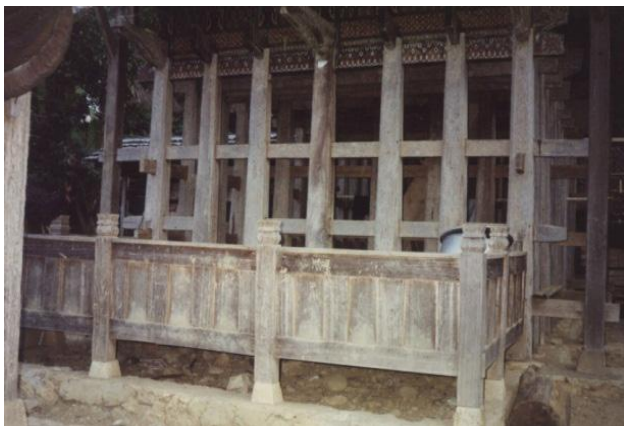
Figure 10. Tongkonan Kesu' s front pole totaling seven, and in front of the pole there is Tangdo as an intermediate space before going up to the top of the house.
