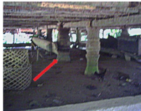
Figure 7. The Andiriposi in the middle of the traditional house in Kondoruba' appears larger than the other pillars (source: Authors' research results).
