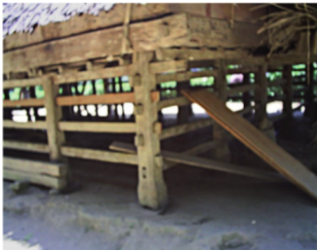
Figure 6. The main pillars of the traditional house in Kaju Bera connected to one another by narrow beams called pelelen (Source: Authors' research results).
