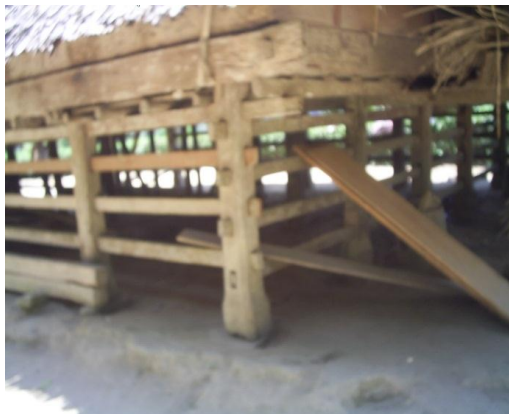
Figure 6. The pillars of the house are connected to one another by thin beams ( Pelelen ) (source: Authors' research results)
