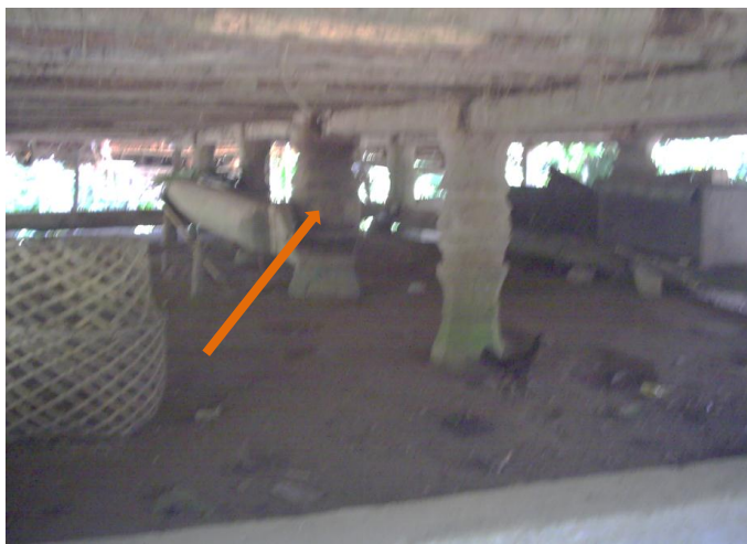
Figure 7. The Andiriposi in the middle of the traditional house in Kondo Ruba' looks bigger than the other pillars (source: Authors' research results).
