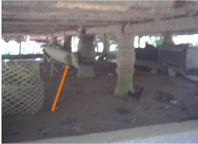
Figure 7. Andiriposi 'in the middle of the house looks bigger than the other pillars decorated with sculptures (Source: Authors' research results)
