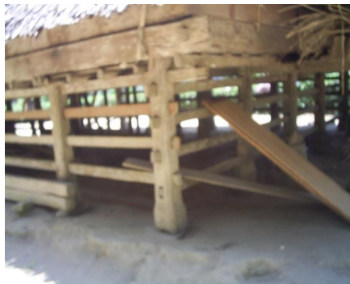
Figure 6. The main pillars of the traditional house in Kaju Bera connected to one another by thin beams called pelelen (Source: Authors' research results).
