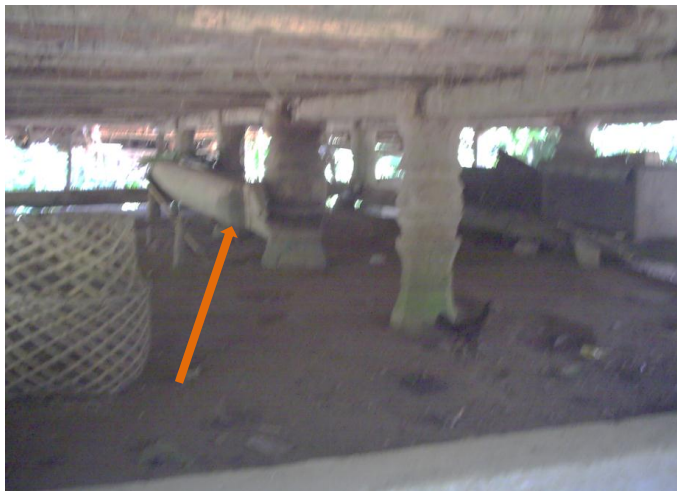
Figure 7. Andiriposi' in the middle of the house looks bigger than the other pillars (source: Authors' research results).
