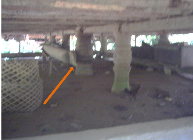
Figure 7. The Andiriposi' in the middle of the traditional house in Kondoruba' looks bigger than the other pillars (source: Authors' research results).
