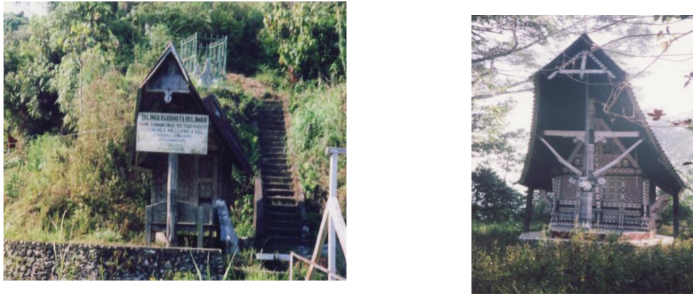
Figure 7: Graves of Batutu ( alang-alang ) type in Messawa and Tabone with roofs using modern structural materials, such as zinc roofs and metal roof tiles
