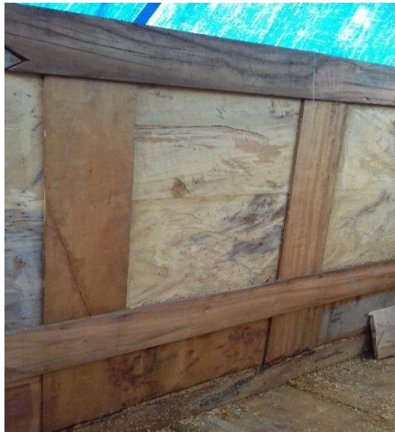
Figure 1. Wall installation (Rinding angin or Rimbang)
