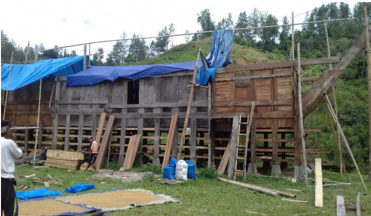
Figure 2. Installation of pole and wall construction has been completed (Banua Sikapu'mi) Source: Research Results
