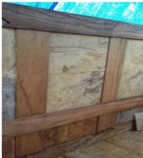
Figure 1. Wall installation (Rinding angin or Rimbang)
